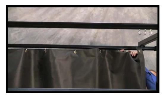
Attach Velcro to outer surface of tracks around entire perimeter. Attach valence around perimeter.
